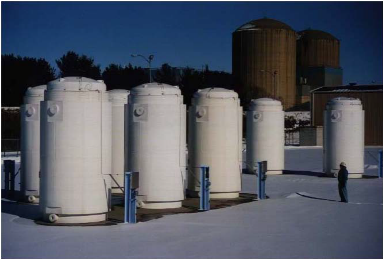
Figure 2-1 Series of Transnuclear (TN)-40 casks at an independent spent fuel storage installation.
